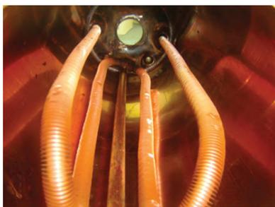
The inside of a Hotpot Calorifier
