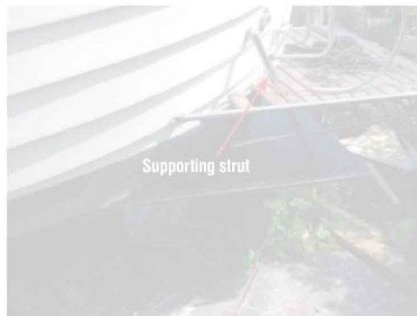
Stainless steel struts help support the outer corners
